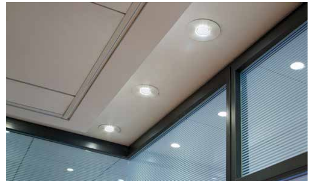
LED lighting retrofit at 888 Seventh Avenue
